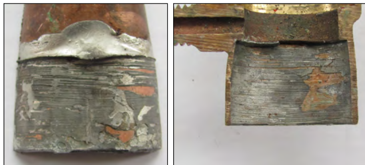
Figure 1: improperly Heated Solder Joint – Brush marks from mechanical cleaning (stainless steel brush inserted in power drill) still evident in soldered surface indicating inadequate heat in the tube surface leading to a lack of solder fill in the capillary space.
