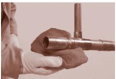
fitting cup and the tube a distance equal to the depth of the fitting cup (Figure 12, position 3). Again, preheating the circumference of the assembly as described above, with the torch at the base of the fitting cup (Figure 12, position 4), touch the solder to the joint. If the solder does not melt, remove it and continue heating.
