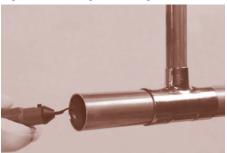
Figure 6. Fluxing: Tube
