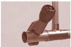
Figure 4. Cleaning: Abrasive Pad
