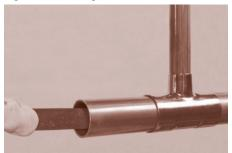
Figure 5. Cleaning: Fitting Brush
