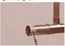
Use care in applying flux. Careless workmanship can cause problems long after the system has been installed. If excessive amounts of flux are used, the flux residue can cause corrosion. In extreme cases, such flux corrosion could perforate the wall of the tube, fitting or both.
